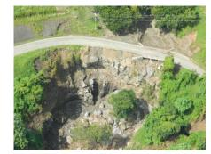
Partial failure of road support along the Windward Highway near Orange Hill cause by overland flow undermining the abutments.
