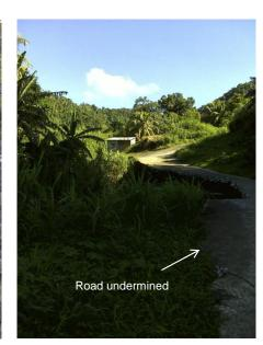
Figure 83: Evidence of landslides and land slippage along the Leeward Highway north of Dark View near N13.28751 W61.24955. Minor road at N13.29209 W61.23801 undermined and damaged.
